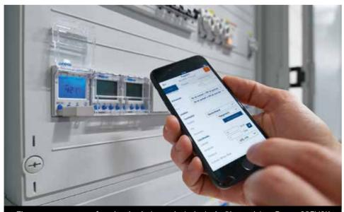
The programs are transferred to the device exclusively via the Bluetooth Low Energy OBELISK top3. This lets you play it safe, since built-in Bluetooth receivers are susceptible to tampering.
